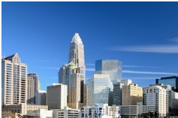
Companies Invest $70 Million to Boost Affordable Housing in Charlotte
